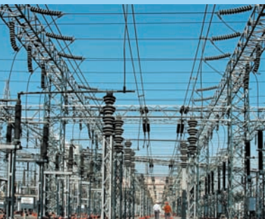
Packaged Industrial PC – Power distribution monitoring
